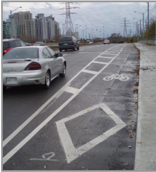
Buffered Bike Lane Toronto, ON
