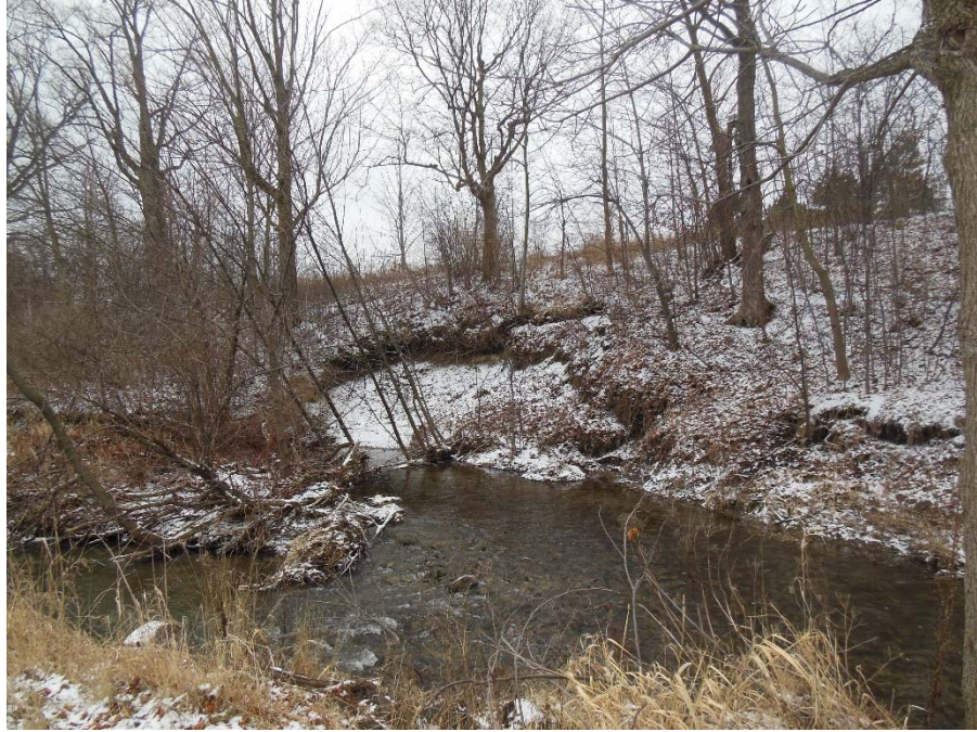
Local sloughing of slope adjacent to Borehole 16-1 looking to the south
