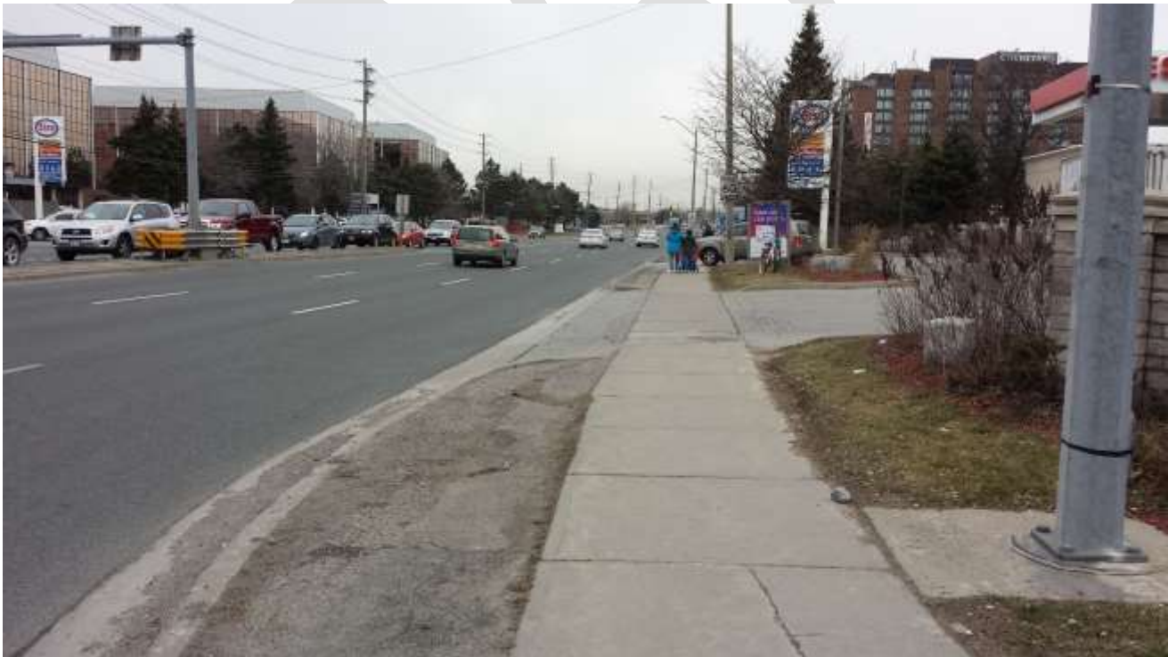
Image 2: A view of disturbances associated with paved roadway/sidewalk/driveway, extant structures, utilities and extensive landscaping.
