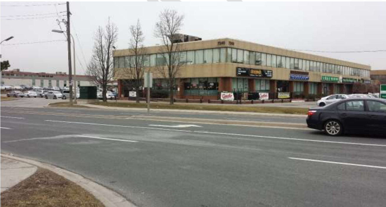
Image 4: A view of disturbances associated with paved roadway, parking area, extant structure utilities and extensive landscaping.
