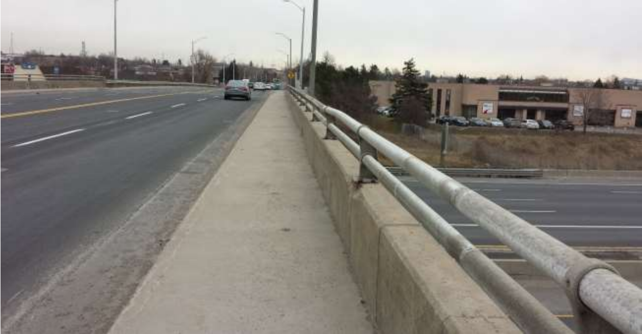
Image 3: A view of disturbances associated with paved roadways/sidewalk, extant structures and utilities.
