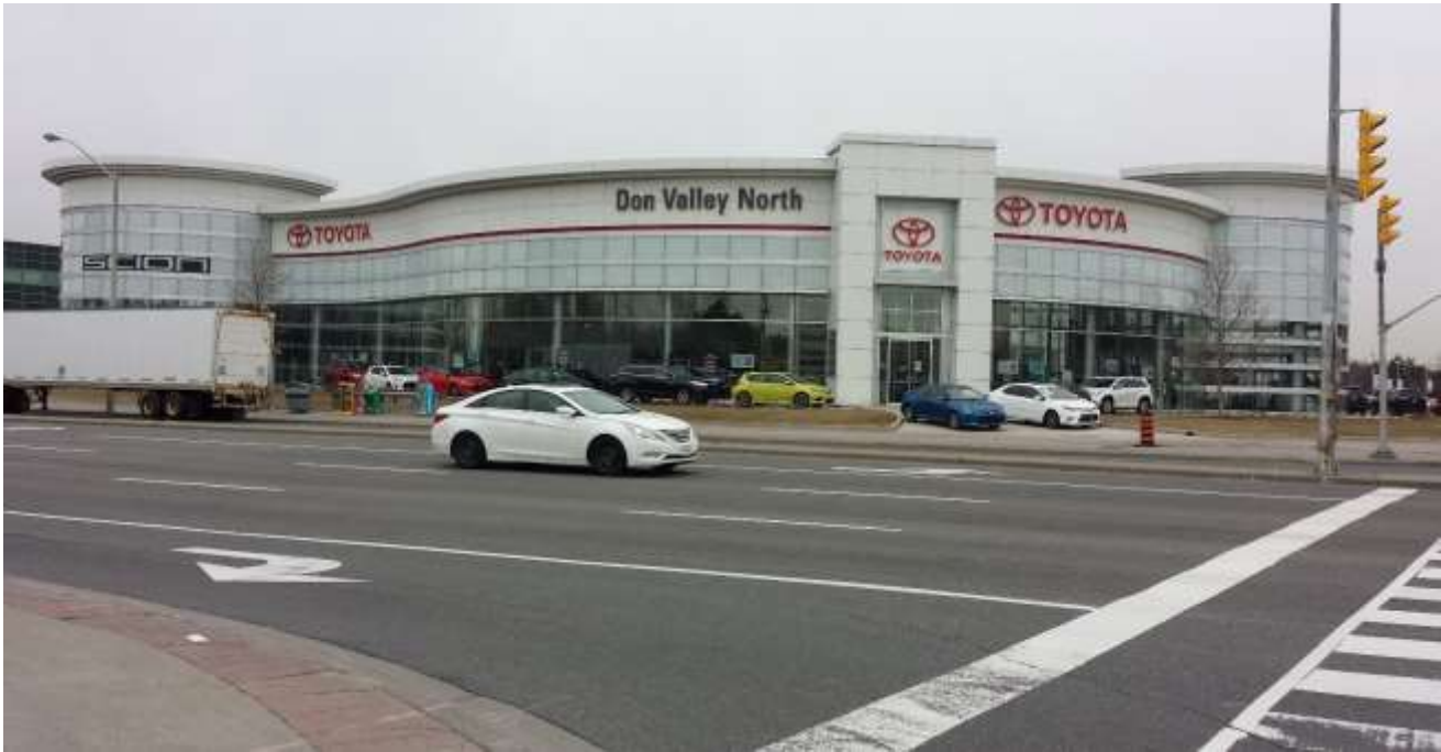
Image 1: A view of disturbances associated with paved roadway/sidewalk, extant structures, utilities and extensive landscaping.
