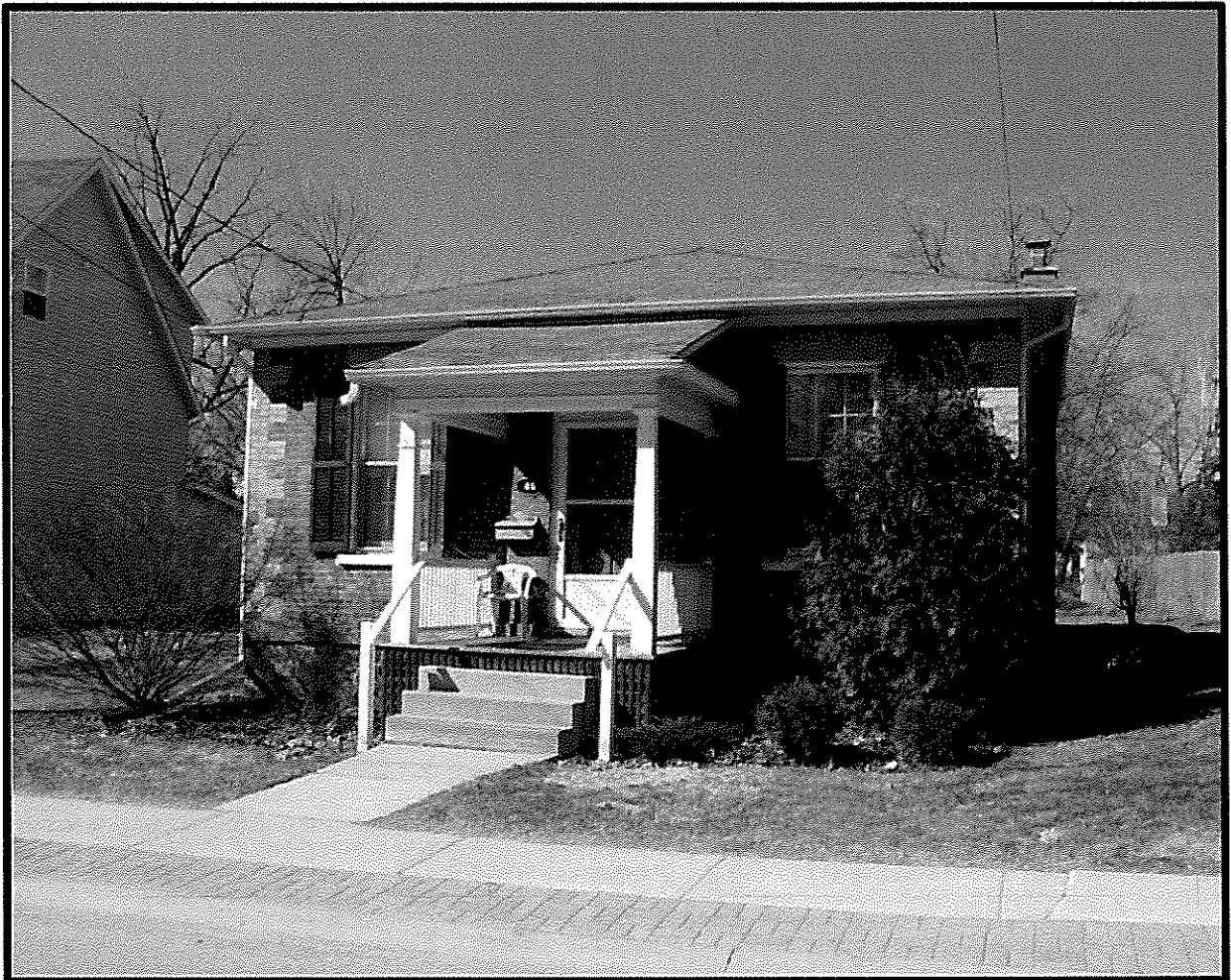
FIGURE 2 – PHOTOGRAPH OF THE EXISTING HERITAGE DWELLING
