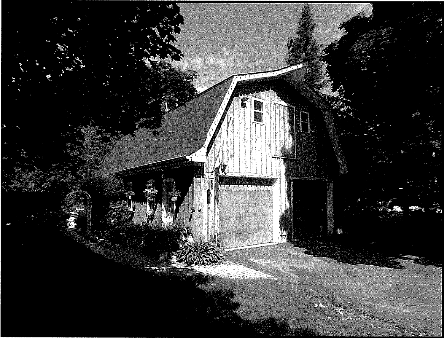
Figure 2- Photograph of the Existing Detached Accessory Building with Existing Secondary Residential Unit.
