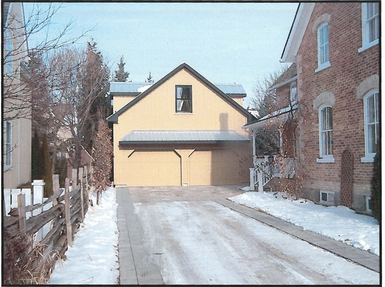
FIGURE 4- PHOTOGRAPH OF THE EXISTING ACCESSORY BUILDING
