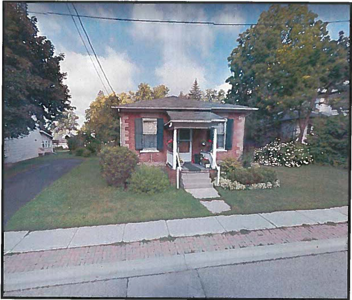
FIGURE 2- PHOTOGRAPH OF THE EXISTING HERITAGE HOUSE
