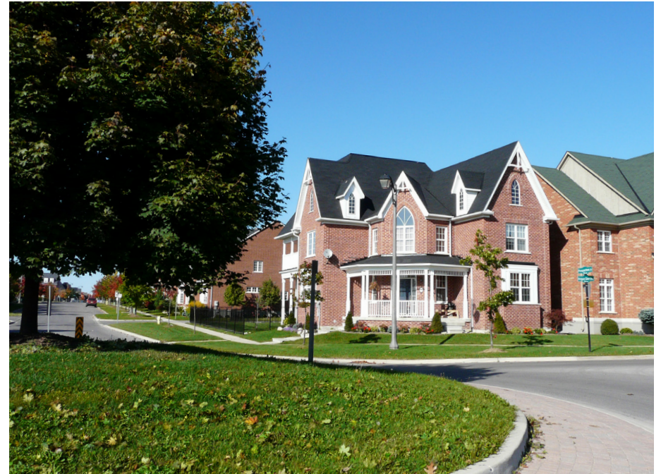
Roundabout homes provide an architectural statement, while addressing two street frontages.
