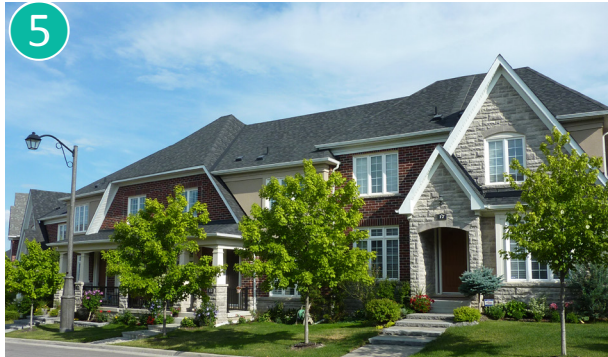
5 Townhouses in Angus Glen are designed with stepbacks and changes in the roofline to break up their massing.
