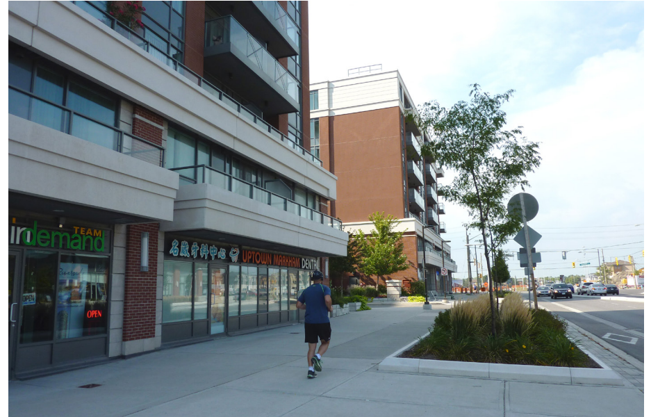
A mixed use edge is proposed along the 16th Avenue edge of the community.
