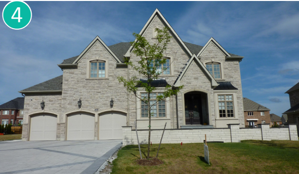
4 Some homes on Glenbourne Park Drive include three car garages and an accentuated roofscape.
