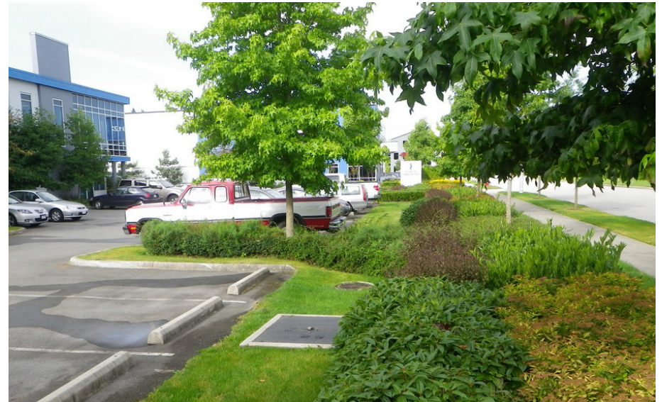
Examples of rain gardens, to be incorporated in the proposed enclaves throughout the community.
