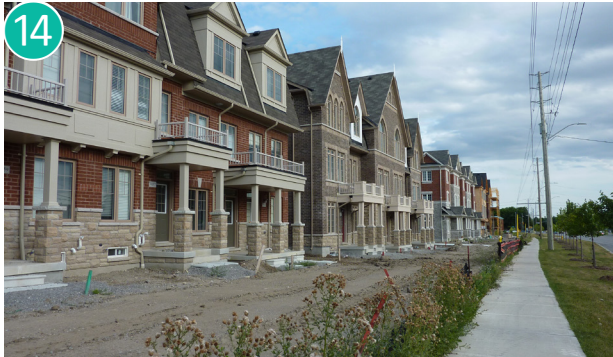
Townhouses under construction in Upper Unionville, east of subject lands.
