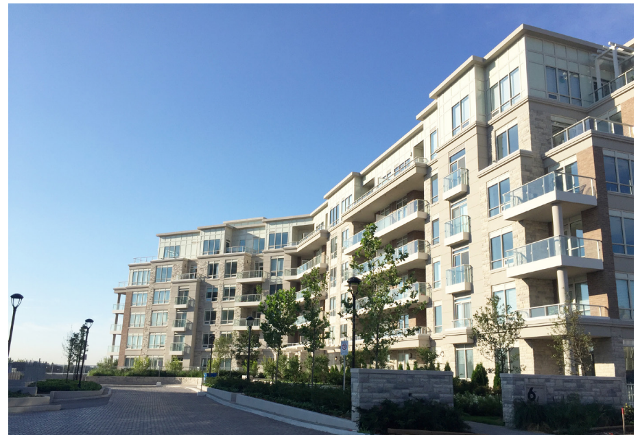
Mid-rise buildings provide additional density, while retaining a human scale and relationship with the street (The 6th Angus Glen).
