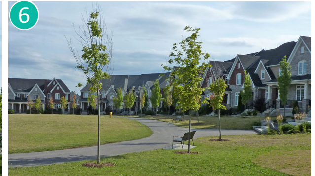
6 Laneway homes front onto the Angus Glen Boulevard Park, creating a strong and consistent streetscape.
