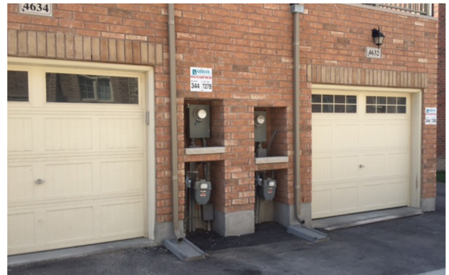
Examples of sensitive integration of utilities to benefit the streetscape.
