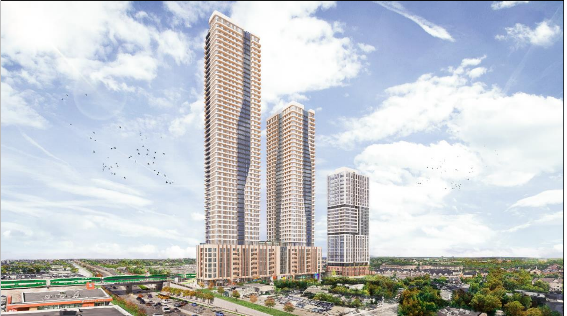
South-east – Metrolinx Bridge and Steeles Avenue Underpass
